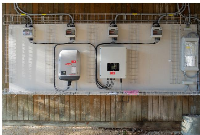
Figure 3: Assembly of the inverters.
