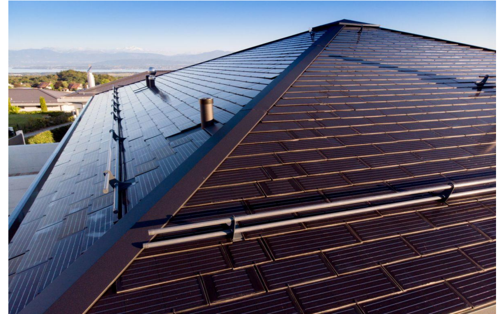
Fig. 1: Chimney shadow on solar roof tiles Fig. 2: Roof structure shadow on PV modules
