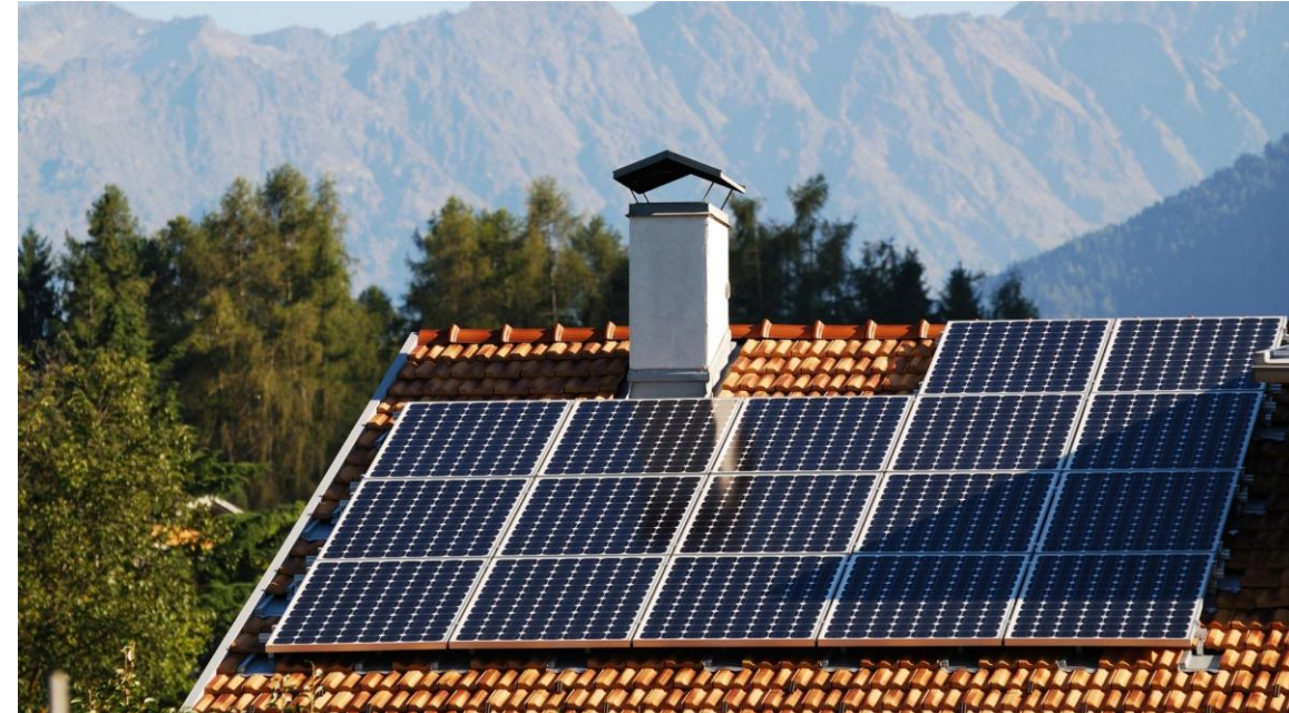
Fig. 1: Chimney shadow on solar roof tiles Fig. 2: Roof structure shadow on PV modules
